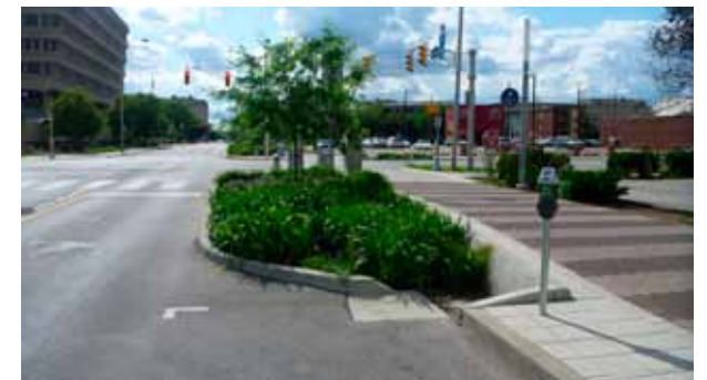
Stormwater Planter at Curb Bump-Out
