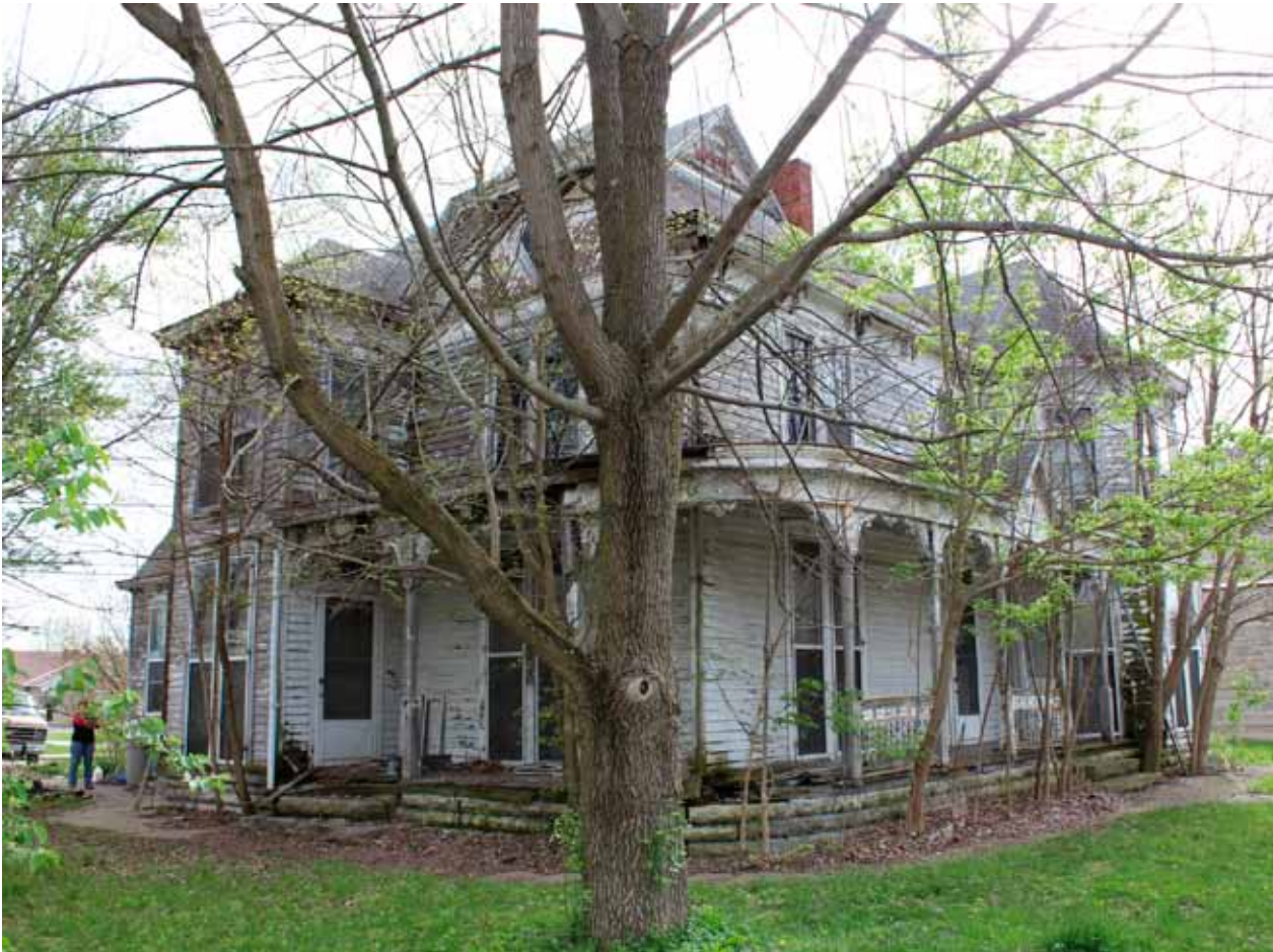
Mulford House on North Street
